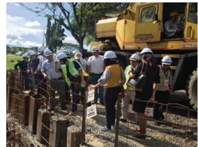
Premier Course: Workshop on Construction Projects in Sarawak -Focus on Risks and Insurance (Visit to Kuching City Centralised Sewage System) 8-9 November 2018
